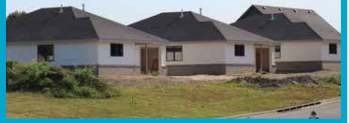
5th Street Sidewalk Project
