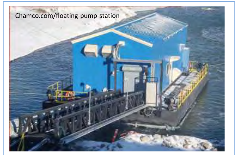
Figure 2-12 Floating Intake Combined with Pump Station
